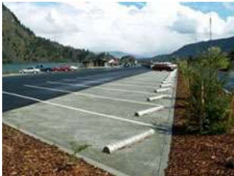
Figure 4-6 – Pervious Concrete Panels
