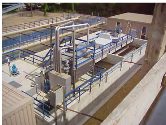
Figure E-3 – Example 25 MGD Enhance High Rate Clarification Treatment Facility
